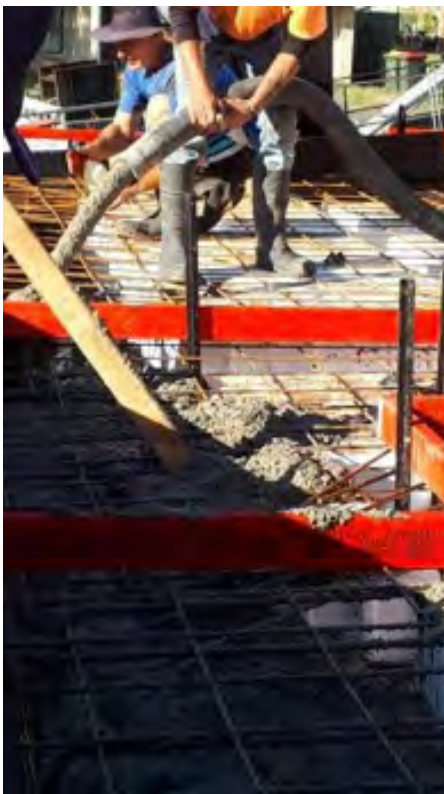
Left: First concrete slab being laid 17th April 2018 - Day 8 on site.
